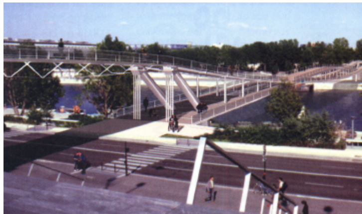
Figura 65 – Passarela Bercy-Tolbiac. (TECHNIQUES ET ARCHITECTURE ,1999)
