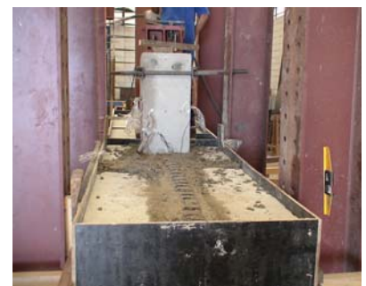
Concretagem entre as lajes
