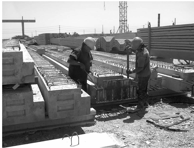
(b) Viga armazenada na T&amp;A (Fortaleza/CE)
