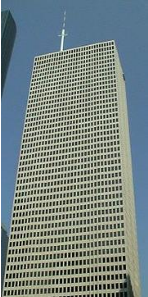
Tube in tube One Shell Plaza 218m -1972 Houston
