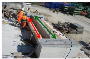
Tensile force in concrete just before first cracking
