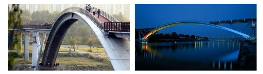
UHPC arch bridge for pedestrians spanning 120m. It consists of 6 precast prestressed segments shaped as double-T beams that are 4.3m wide and 1.3m deep. The deck is 30mm deep and has transverse ribs every 1.225m.
