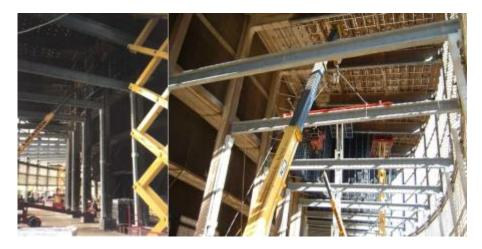
UHPC solution was selected to upgrade the Cattenom power station cooling towers. Specifications were clear; they required a building **material that could withstand physicochemical aggressions** (run-off water, sulfates, thermal gradient & freeze/thaw cycles) for the beams and girders providing the support structure of the heat exchange building.
