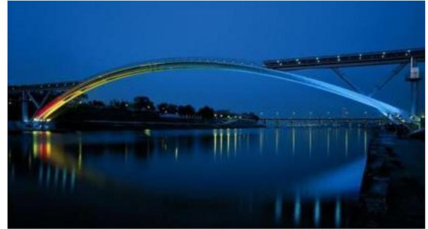
UHPC arch bridge for pedestrians spanning 120m. It consists of 6 precast prestressed segments shaped as double-T beams that are 4.3m wide and 1.3m deep. The deck is 30mm deep and has transverse ribs every 1.225m.
