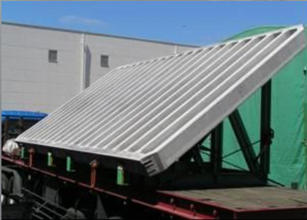
7000 prestressed slabs assembled by post-tensioning to make the runway of airport extension over the sea (50 000 m<sup>2</sup>)
