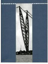
Pier Luigi Nervi (1891-1979) The hall of the Turin Exhibition Center "is formed by the assembly of prefabricated elements in ferrocement, assembly completed by reinforced concrete ribs, cast in situ, and arranged in the hollow and the top of the wave". **Page 104, in Savoir Construire - Nervi**
