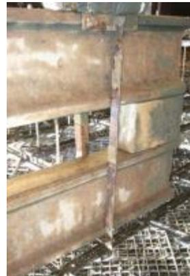
Test samples taken in 2008, (after ten years of being subjected to a stream of pure water at 35°C) showed that the UHPC material had no degradation of mechanical properties when compared to the initial measurements taken.
