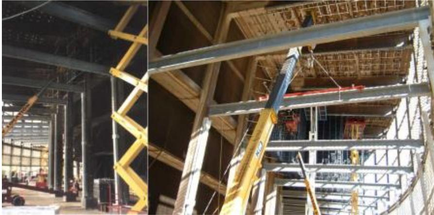
UHPC solution was selected to upgrade the Cattenom power station cooling towers. Specifications were clear; they required a building **material that could withstand physicochemical aggressions** (run-off water, sulfates, thermal gradient & freeze/thaw cycles) for the beams and girders providing the support structure of the heat exchange building.
